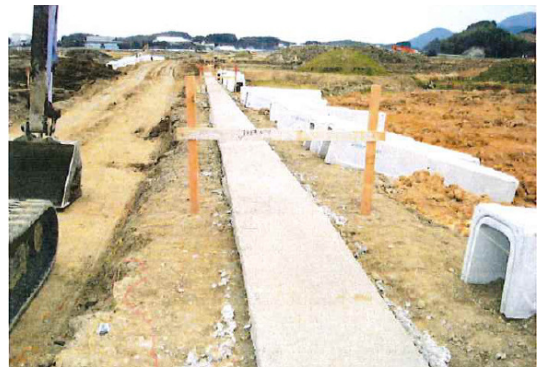
ช) Side ditch base concrete
