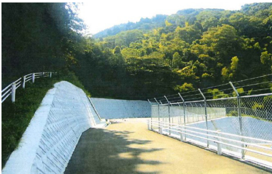
ก) Backfilling concrete and top end concrete
