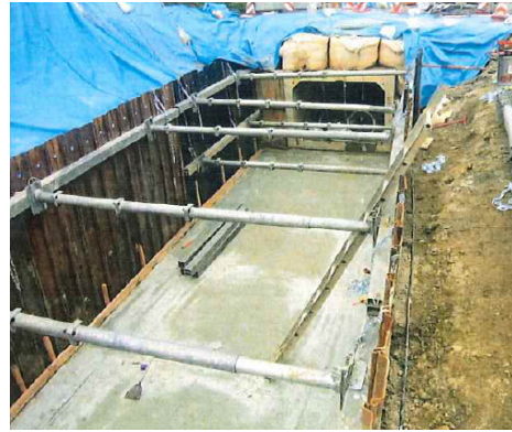
จ) Box type culvert base concrete
