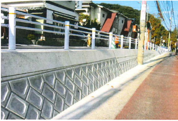
ง) Gravity type retaining wall, backfilling top end concrete
