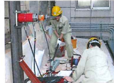
On-site test regarding (Performance test of external wall)
