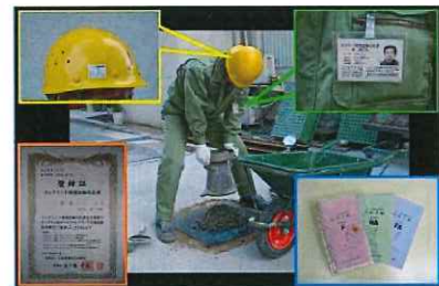
Certificate and license card of skillful concrete worker
