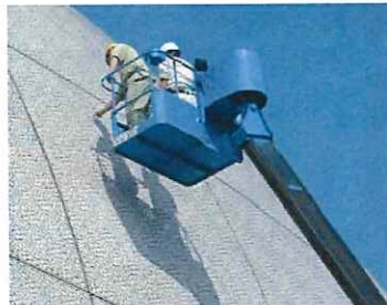
Field investigation (Investigation of external wall)
